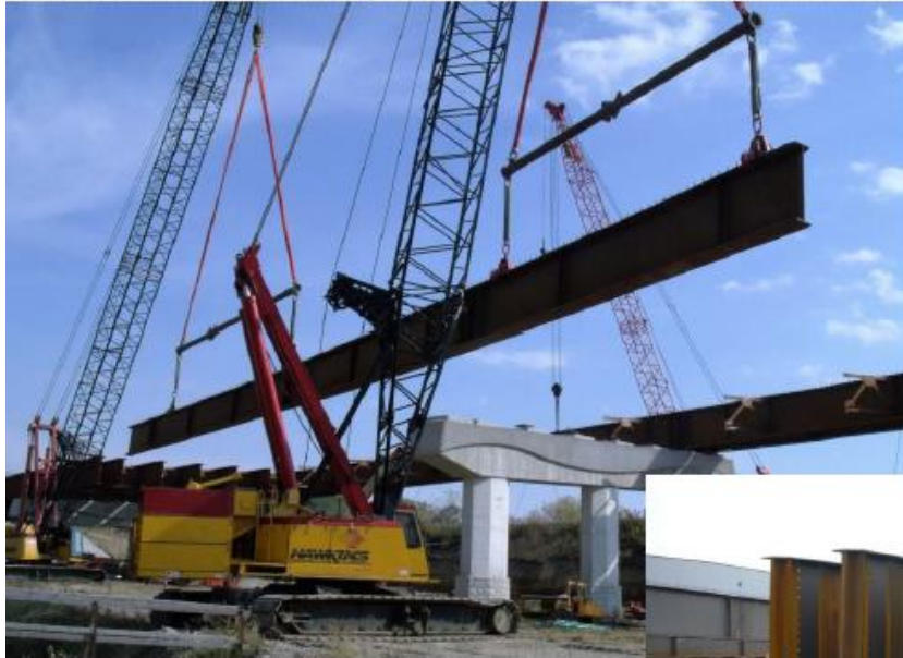
Beams in Bridges-Construction and installation
